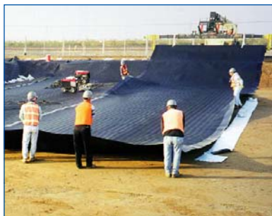
Workers position a piece of thick, plastic liner over the compacted soil base. This piece of plastic liner will be welded to the adjacent pieces of plastic liner.
