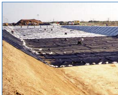
This ash landfill "cell" under construction shows compacted soil base, a thick, plastic liner, and a drainage layer. The berm is designed to contain water to be collected for safe disposal.
