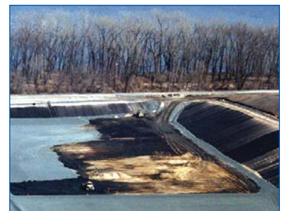
Construction of this ash landfill cell is complete and the landfill has begun to receive ash.
